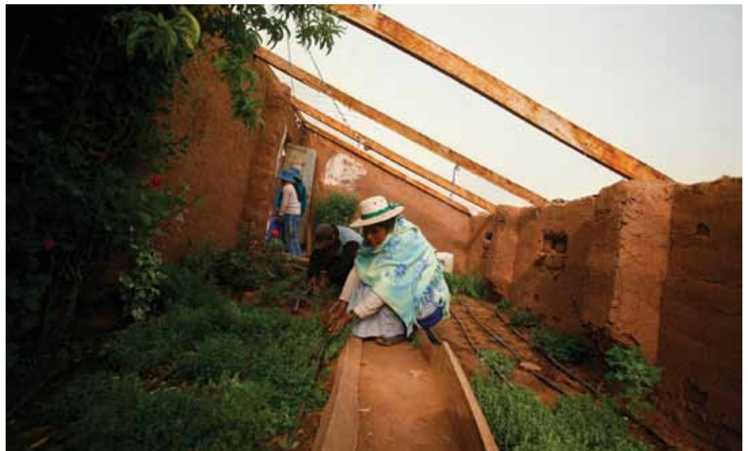
Drip irrigation system to conserve water in an arid area of Bolivia (CAFOD)
